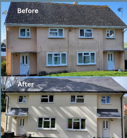
In Dartmouth, Devon, 42 homes have had replacement roofs put on, new soffit and fascias fitted with new rainwater pipes and guttering, new windows and doors, external wall insulation and new canopies. New external lights have also been put in place and pea shingle has been placed at the front as a rain protector.
