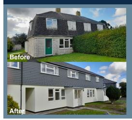
DIO is starting the fourth phase of work at Culdrose (with the first three already completed). The project has helped transform the poorly insulated and non-traditional houses in Culdrose to get rid of 'cold spots' by replacing important features like doors and windows. So far, many of the houses have seen major improvements which include building new bathrooms, replacing boilers, rewiring electrical systems, adding loft insulation, and upgrading the heating system.
